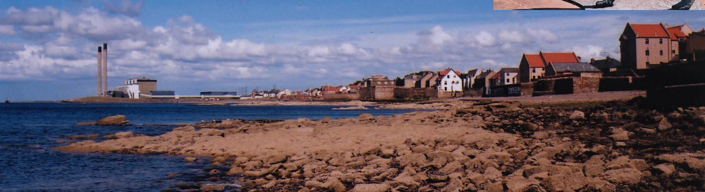
Prestonpans looking at Cockenzie Power Station
