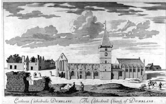
Below Left: Engraving showing Dunblane Cathedral from the south west, 1821
