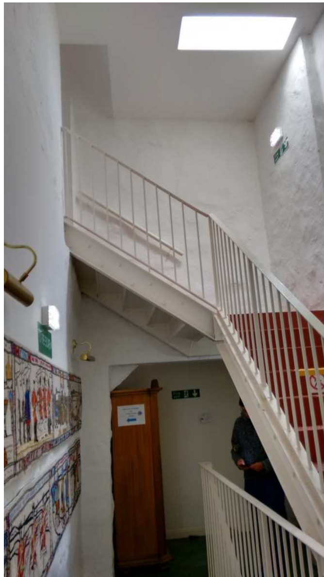
8. Skylight allowing ultraviolet radiation from daylight stream on the Tapestry panels.
