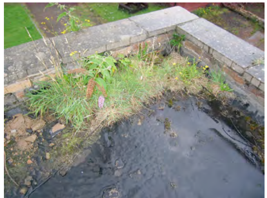
Detail of roof showing failure of asphalt and cope
