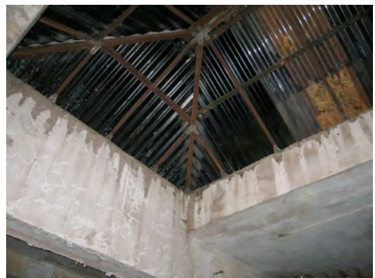
Steel framed roof lantern
