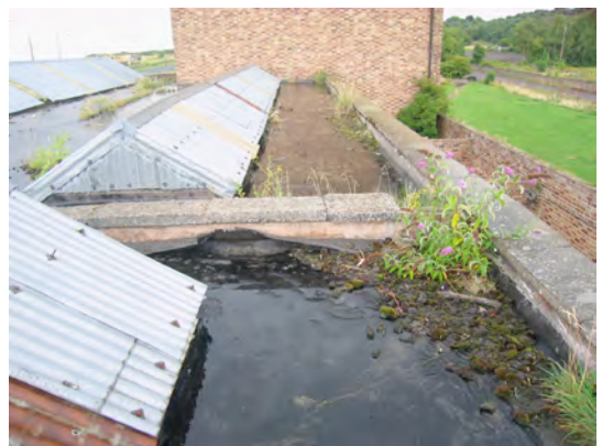
Failing copes, upstand and deck to main roof
