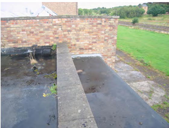
West canopy roof and crack to brickwork
