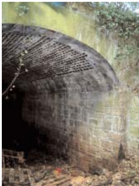
Figure 17: Another view of the tunnel, and in particular the fine masonry work. © A Ralton, 2004.
